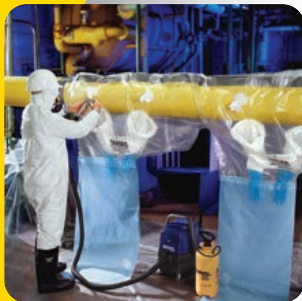
QT14 It safely encloses pipe diameters from 10" to 14".
