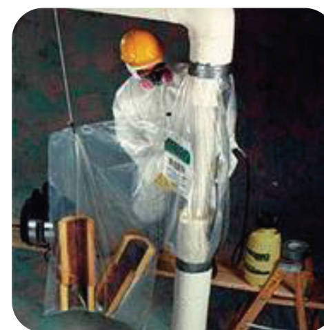
V10 This Avail glovebag sets the industry standard for efficiency on vertical pipe diameters up to 10". Each bag measures 60"x84". An offset debris area moves the weight and bulk away from the work area. One arm set, and ports per chambers, 6-mil construction.
