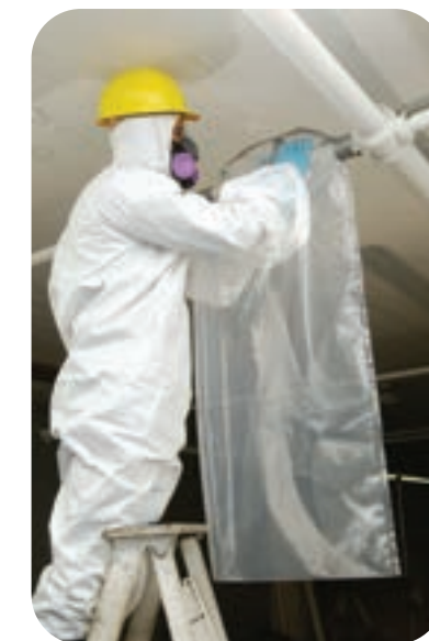
M6 The M6 is for repair and maintenance operations where the work is on small sections of insulation or gasket replacement. For pipe diameters up to 6". Each chamber measures 22"x60" with one arm set with opposing glovesleeves, 6-mil construction.
